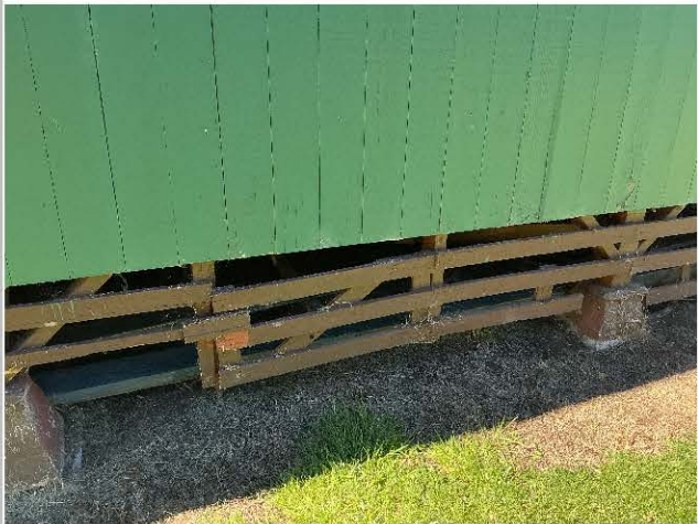
Polipoli-Spring-State-Recreation-Area_Cabin-Structural Repairs and Painting_Remove and Replace Rotted Post
