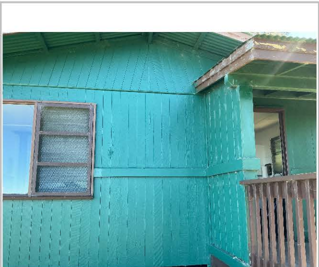
Polipoli-Spring-State-Recreation-Area_Cabin-Structural Repairs and Painting_Prep and Paint
