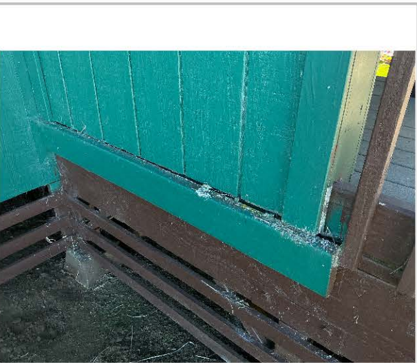
Polipoli-Spring-State-Recreation-Area_Cabin-Structural Repairs and Painting_Remove and Replace Rotted Boards and T&G Siding
